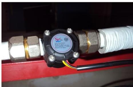
**Fig. 8 – Installation of volumetric flow meter to the panel (DV1)**
