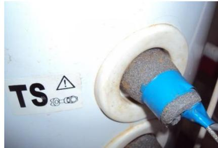
Fig. 5 - Installation of thermal detector to the boiler inlet (S2)
