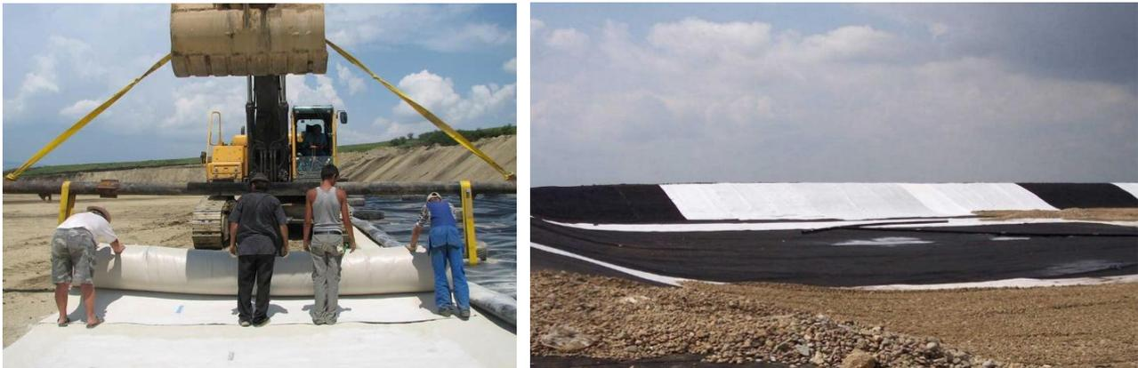
**Fig. 1 – Examples of geomembrane and protection geotextile utilisation in the construction of waste landfills**
